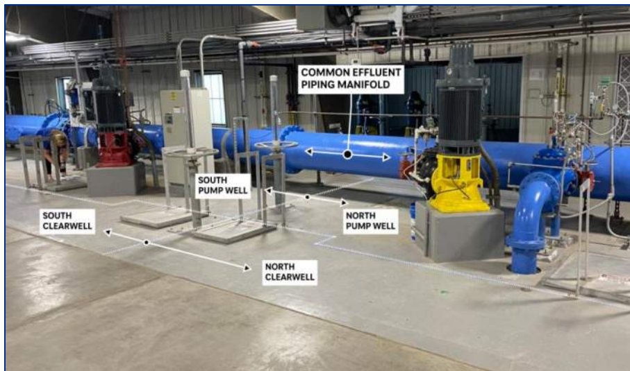
Figure 2.2 Operating Floor with Wet Well Delineation
